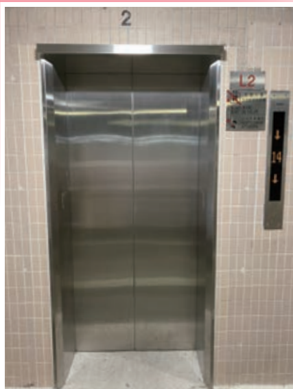
升降机新外门和楼层显示器 New lift landing door and floor indicator
